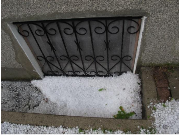
Bailing out water and hailstones
